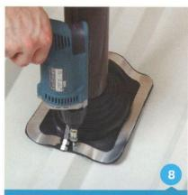
Use fasteners to complete sealing. For installation, fastener spacing may not exceed 1.5" (38 mm).
