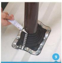
Additional sealant may be applied between the flashing and the pipe.
