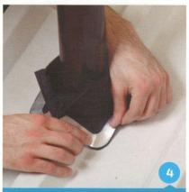
Press Master Flash® Multi down, bending it to conform to roof profile or roof irregularities. A blunt tool will help press the flashing into tight roof angles.
