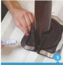
Apply sealant between the base, roof and at the top of the flange.
