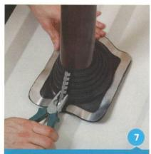
Tighten the stainless steel clamp.
