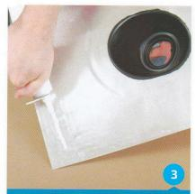
Apply sealant on the bottom side of the metal base.
