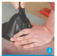
Finish the diameter by adjusting the flashing by hand.
