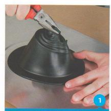
Use pliers to pull the tab for the correct pipe size.
