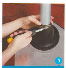
Apply a stainless steel band to assure tight fitting of the flashing against the pipe.
