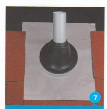
Install the tiles at the side of the flashing.
