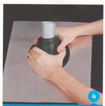
Slide the flashing down the pipe.
