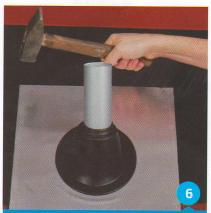
Fasten the metal base using nails and a hammer.
