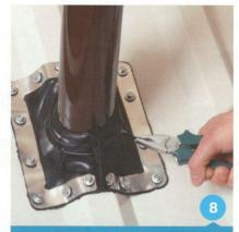
Put the cable through the hole to assure tight fitting.
