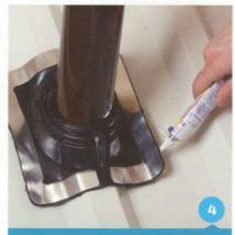
Apply sealant between the base, roof and at the top of the flange.
