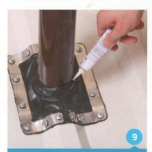
Additional sealant can be applied between the flashing and the pipe.
