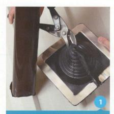
Select an appropriate Master Flash® Retrofit. If necessary trim opening to the pipe diameter.
