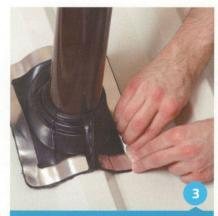
Press Master Flash® Retrofit down, bending it to conform to roof profile or roof irregularities. A blunt tool will help press the flashing into tight roof angles.
