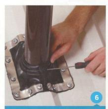
Make a hole in the flange to insert a cable tie.
