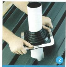
Slide Master Flash® down the pipe (a nonpetroleum base lubricant will ease installation).
