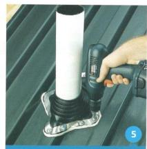
Use fasteners to complete sealing. For installation, fastener spacing may not exceed 1.5" (38 mm).
