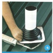
Apply sealant between the base and the roof.
