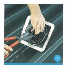
Choose an appropriate Master Flash® with opening at least from 20% to 30% smaller than pipe diameter. If necessary trim opening to 20% smaller than the pipe diameter.
